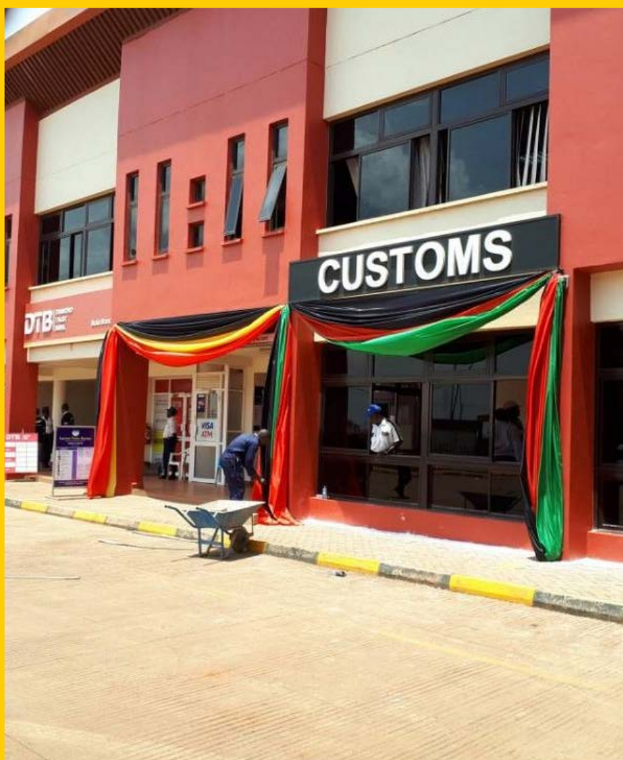
Revamped border crossing in Busia between Uganda and Kenya
